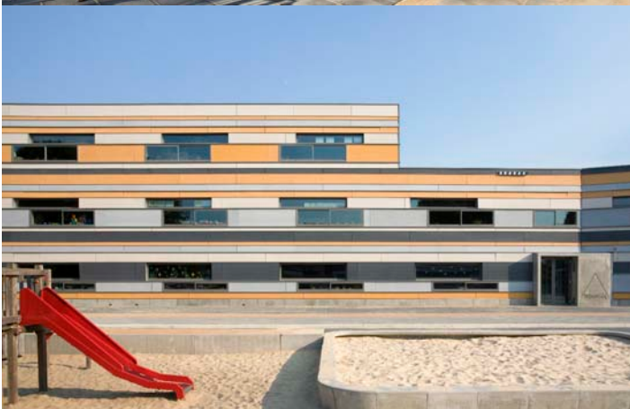
Brede School MFA Eninver Almelo architect: Vera Yanovstchinsky Architecten
